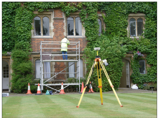
Fig. 3. Surveying the wall using GPS.
