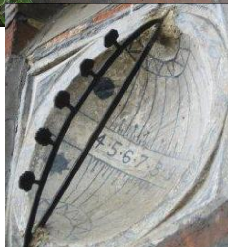
Fig. 2. (Top) The Five Elms pub at Weedon; (centre) the scaphe dial; (bottom) close-up of the gnomon.
